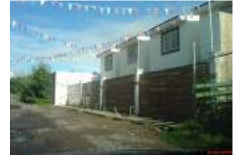
Condominium Villas de Guadalupe Construction of 8 homes Zapopan, Jalisco
