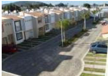
Villas de Santa Mónica Construction of 104 homes Zapopan, Jalisco
