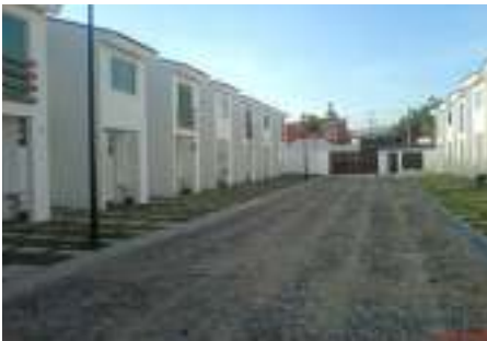
Condominium Santa Lucía Construction of 29 homes Zapopan, Jalisco
