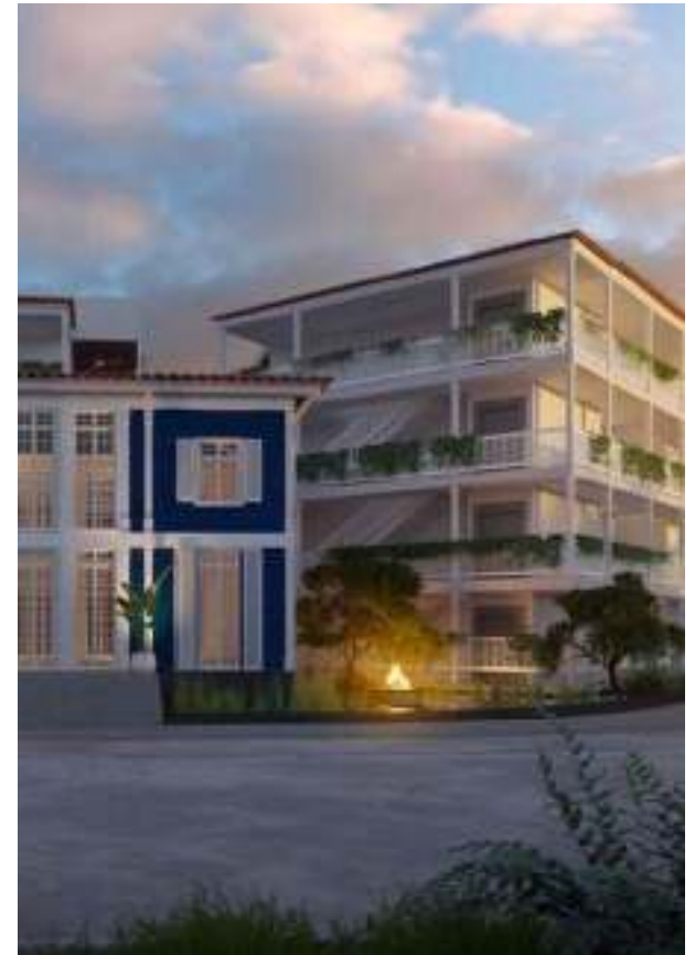
Blue House Residences Condominium of 26 apartments in Puerto Aventuras, Quintana Roo. In Progress
