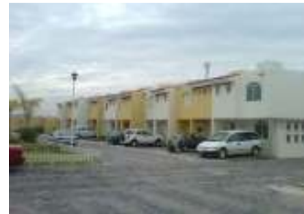
Housing Development Santo Tomas Construction of 53 homes Zapopan, Jalisco
