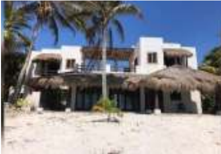
Remodeling of Tankah House Tulum, Quintana Roo In Progress
