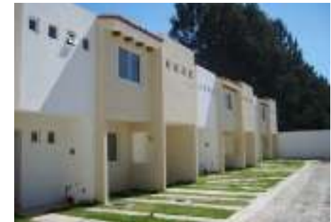
Condominium San Francisco Construction of 16 homes Zapopan, Jalisco
