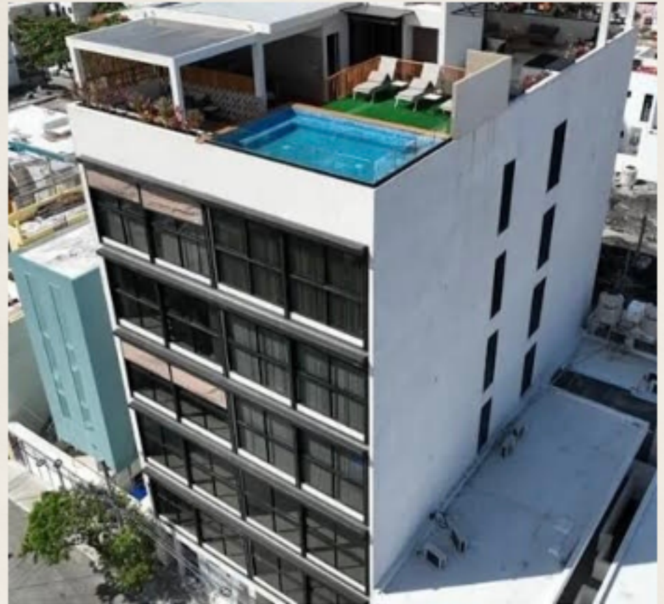
Tower 25/Kiin Tower (Construction)
