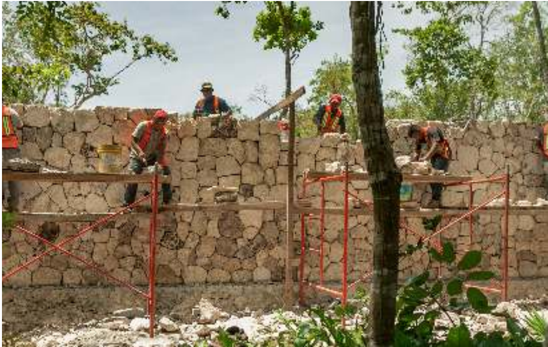
Perimeter wall - Handmade local limestone
