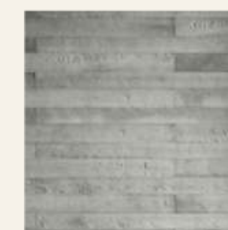
3. Wall Concrete decking Building Front
