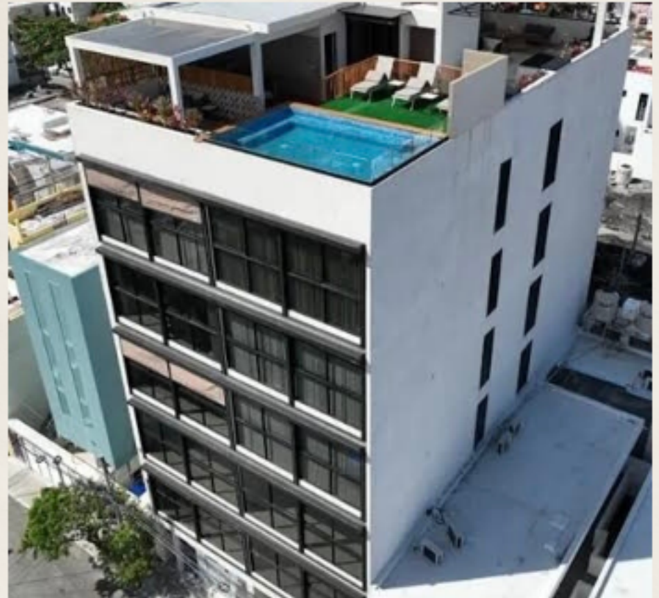
Tower 25/Kiin Tower (Construction)
