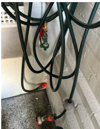
Universal tap adapter and hose with controllable nozzle
