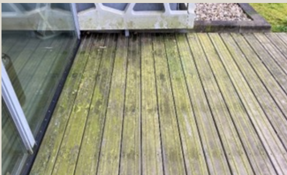
Example of a deck in worst application situation of north facing, shaded and not cleaned for 4 years. Notice the staining is also affecting the concrete façade panel in this extreme situation.
