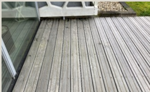
Example of a deck in worst application situation of north facing, shaded and not cleaned for 4 years. Notice the staining is also affecting the concrete façade panel in this extreme situation.
