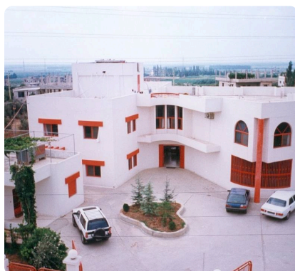
The Halba Center in Akkar, 1996
