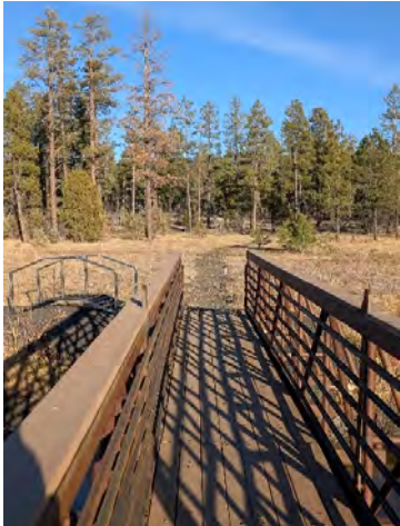
The Rollover Gate waiting to be installed
