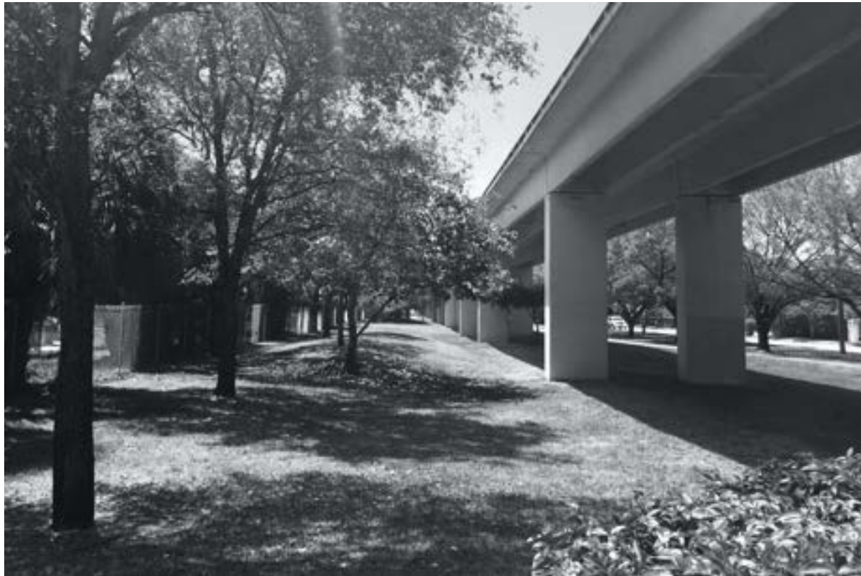
Previous conditions near Vizcaya Station
