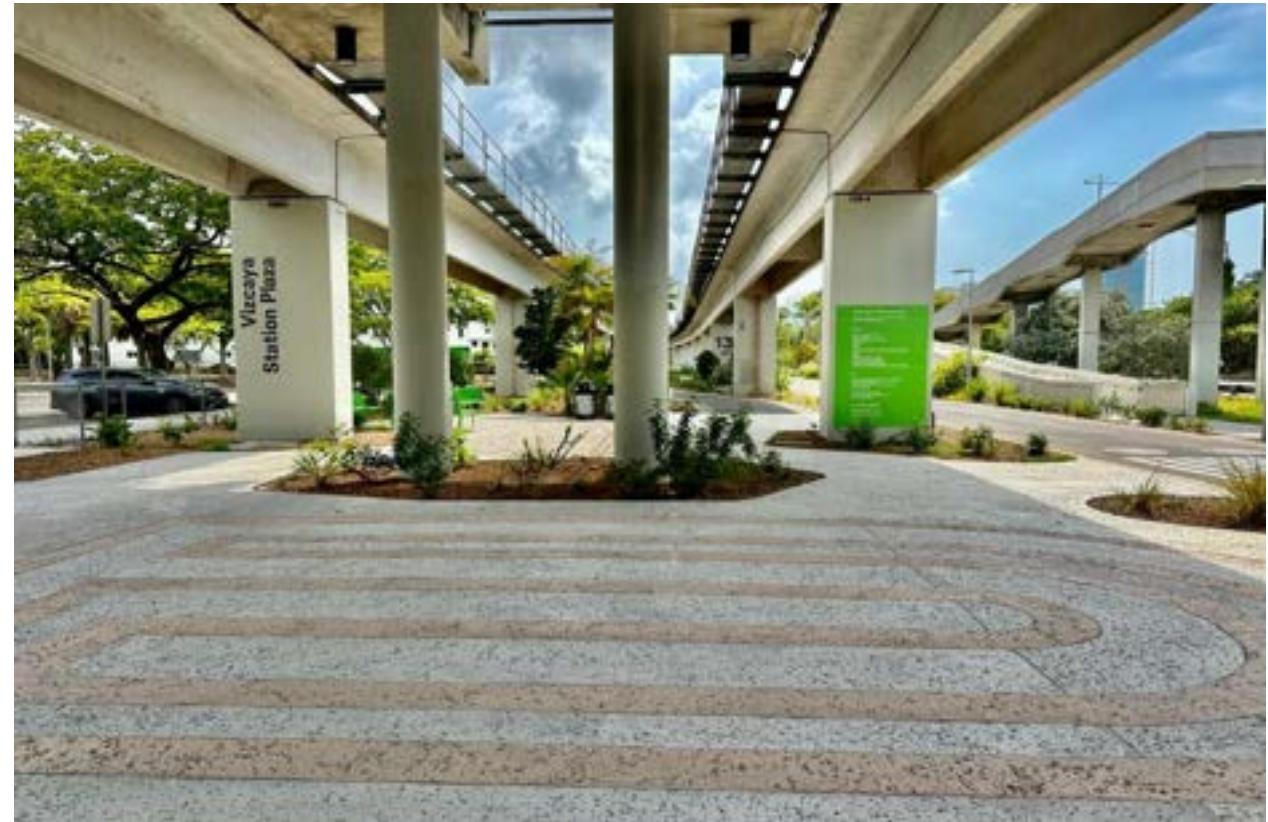
Current conditions in Vizcaya Station
