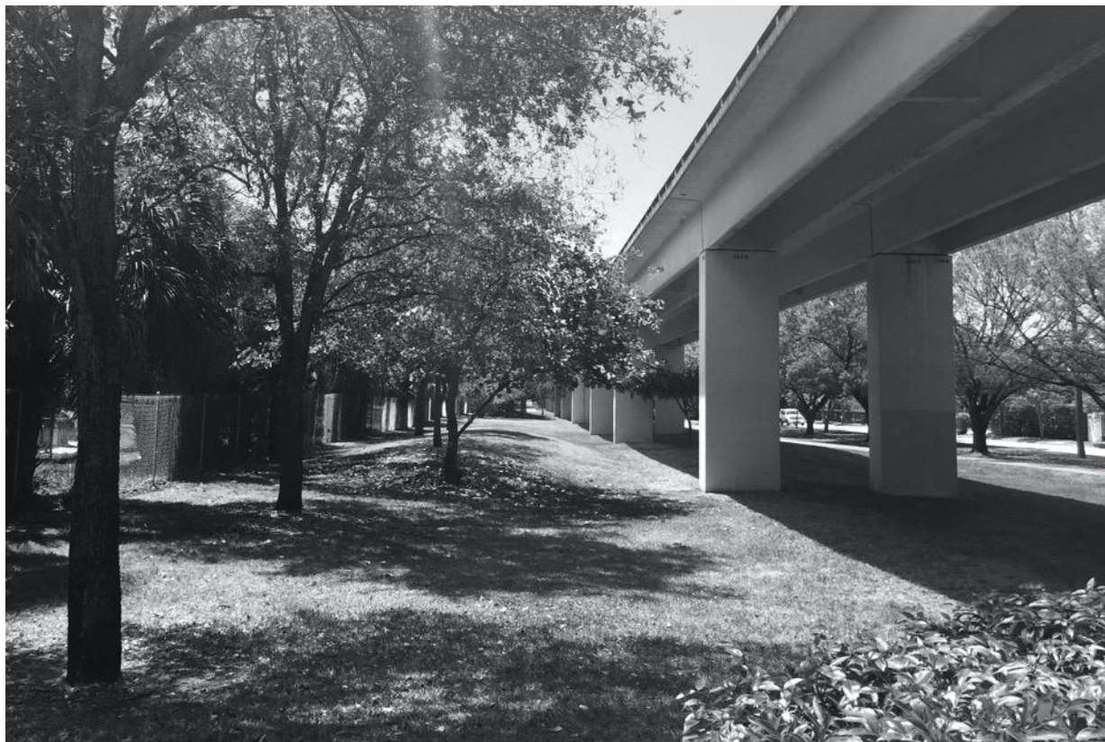
Previous conditions near Vizcaya Station
