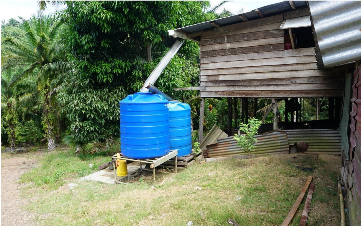
Figure 2 Rainwater harvesting in Kg. Pendising
