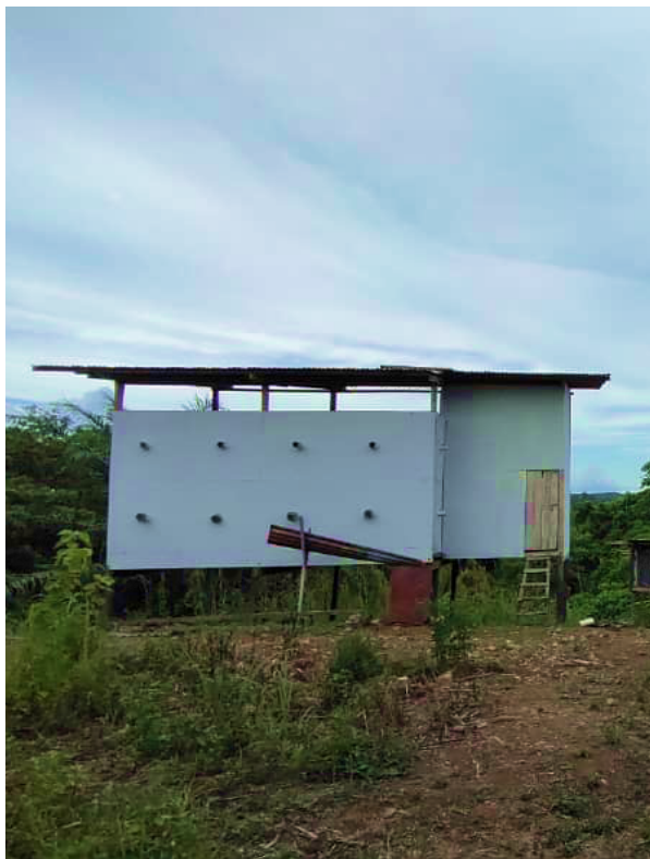
Figure 9 Some of the swiftlet houses that belong to the villagers (private owned)
