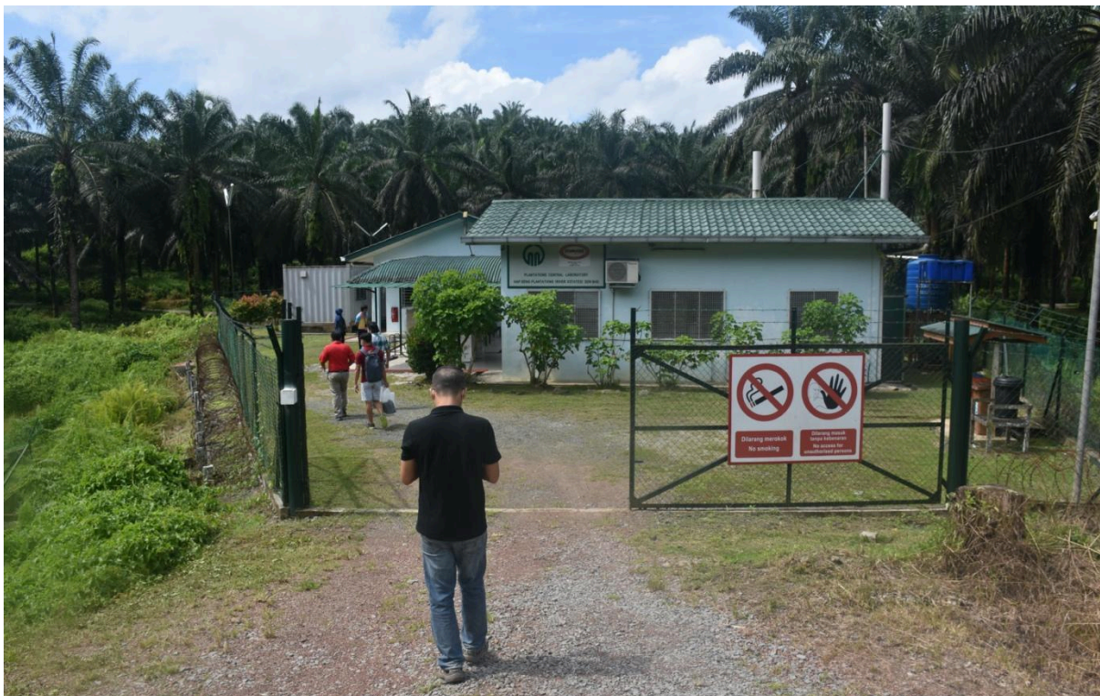
Figure 22 Plantation Central Laboratory Unit in PCO, Hap Seng
