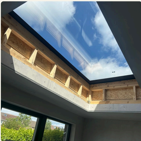
Part-way through: a rooflight framed and glazed, before the ceiling is finished.
