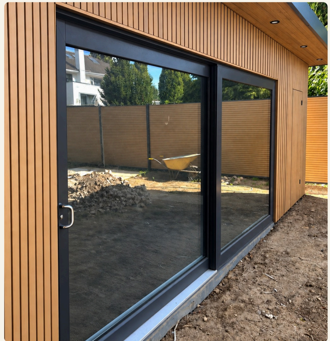
Composite cladding and aluminium sliding doors on one of our rooms.
