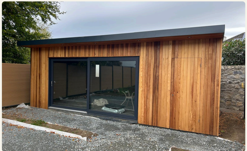
The slab from the previous page, with its finished timber-clad room.
