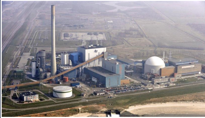
Coal fired Boilers and steam turbines (1996)
