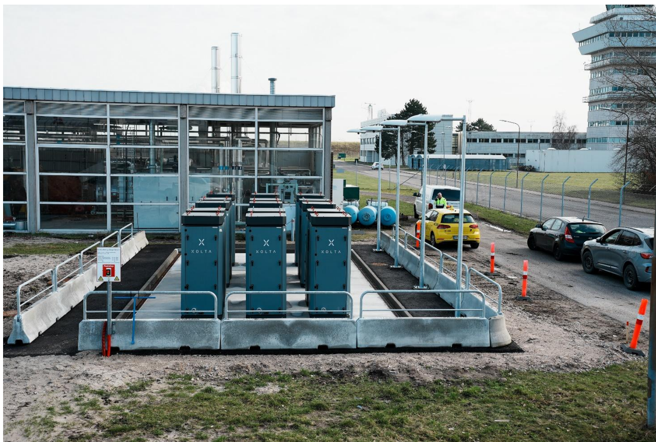
Figure 27 – The final installation of the BESS consisting of 15 racks from Xolta.
