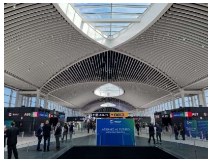
Figure 10 - New Pier A
