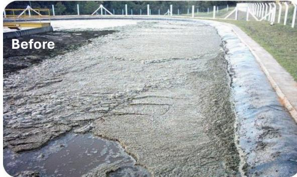
90,000 animal per day slaughterhouse with excessive surface FOG buildup and odors in treatment tanks. Treatment capacity of 2,250 cubic meters per day with 8-day retention time. Low efficiency in reducing BOD with final effluent at 860 mg/L.
