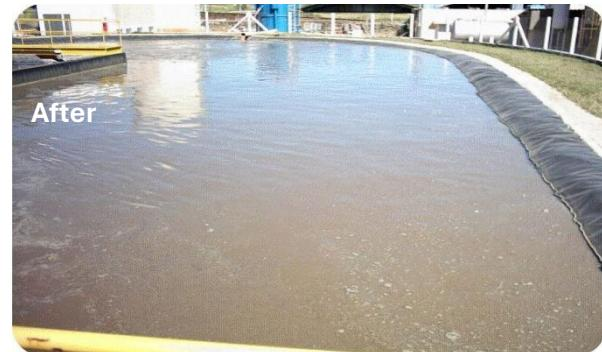
Odors and surface fats, oils and grease (FOG) were eliminated. BOD reduced from 860 mg/L to 121 mg/L in effluent. Efficiency increased from 55% to 86% within 90 days of treatment.
