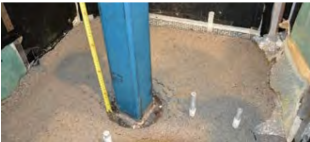
Pavement with geogrid
