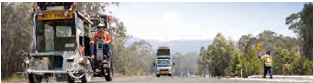
Road Tek Line-marking machine convoy Image Source: Queensland Department of Transport and Main Roads (TMR).
