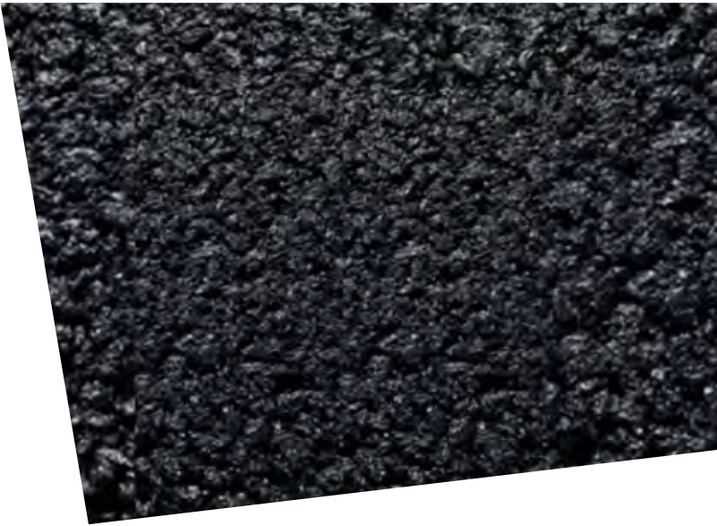
Finished crumb rubber modified gap graded asphalt surface Image Source: ARRB
