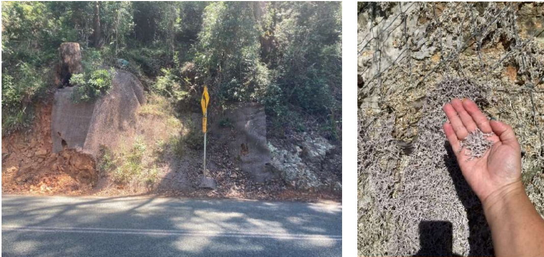
Figure 4.8: Turf reinforced matting crumbling as a result of exposure to the elements
