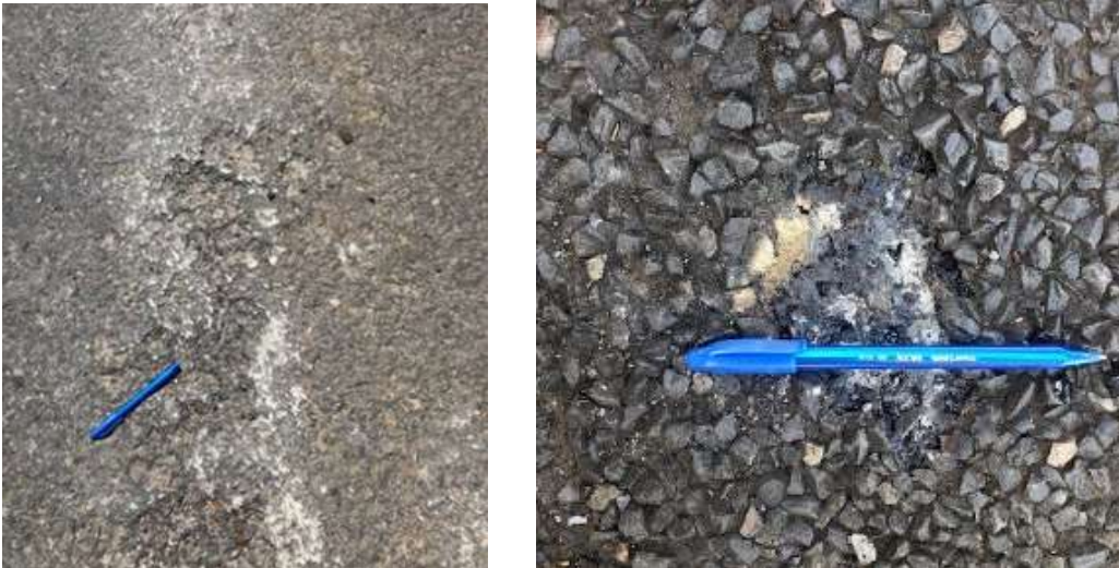
Figure 4.7: Damage to pavement materials from bushfires (left image: asphalt; right image: sprayed seal,)
