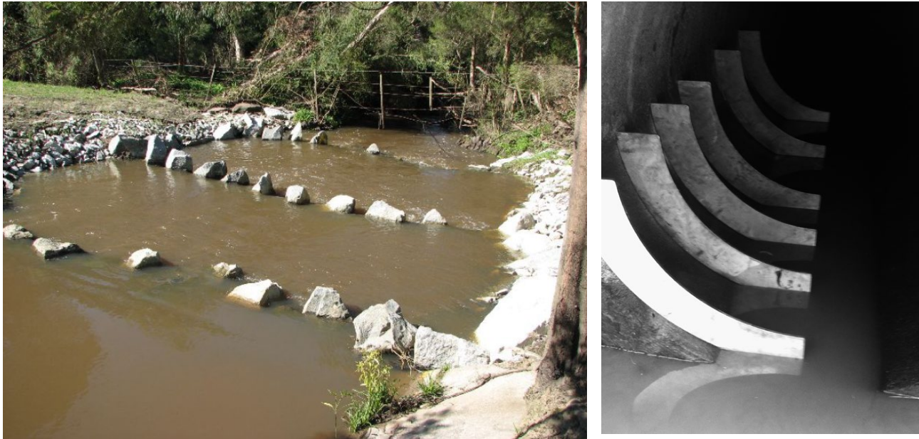
Figure 2.15 Cardinia Creek rock ramp fishway (L) and pipe culvert baffles (R)
