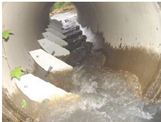
Figure 2.12 Corner 'quad' baffles
