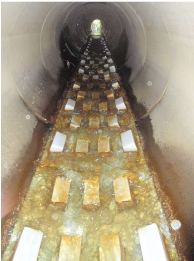
Figure 2.23 Pipe culvert spoiler baffles under low flow conditions
