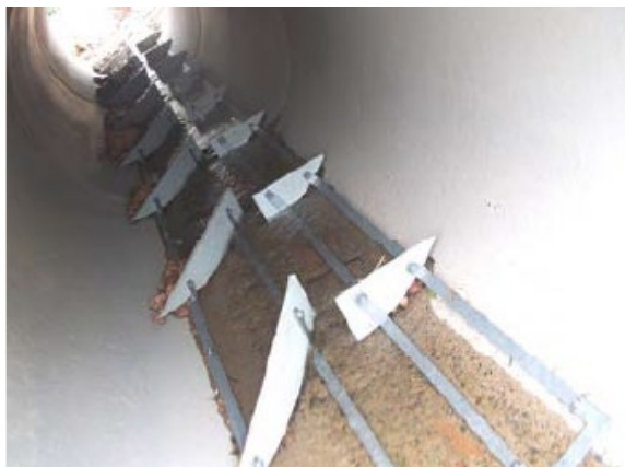
Figure 2.11 Offset baffles
