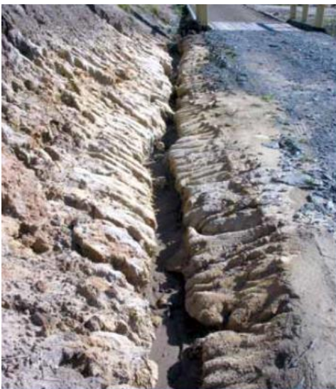
Figure 2.13: Example of table drain constructed in dispersive soils
