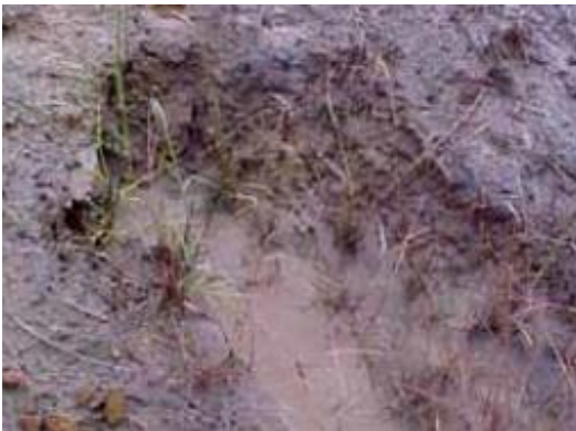
Figure 3.5: Example of spew holes or sediment fans
