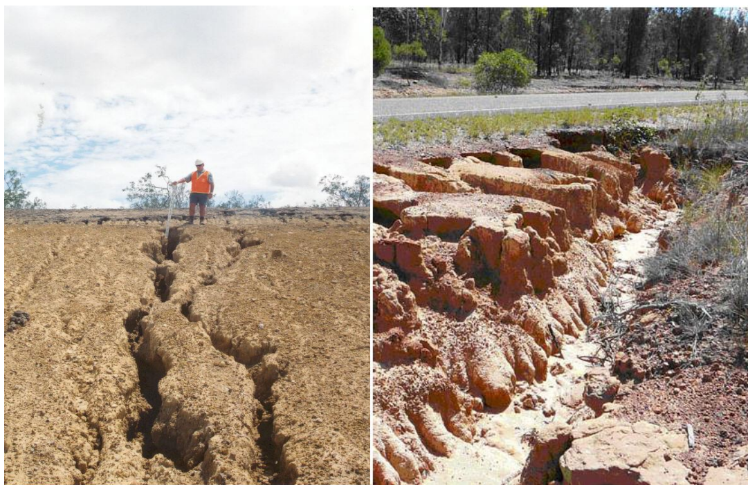
Figure 1.1: Examples of erosion due to dispersive soils
