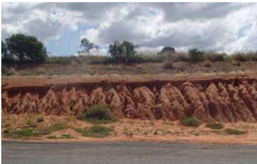
Figure 2.8: Image of dispersive sub soils exposed on a cut batter showing the stable topsoils overlaying the dispersive subsoils
