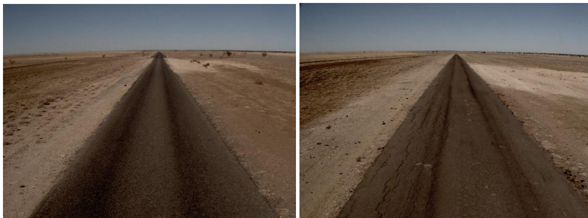
Section 5803: chainage 18.7 km to chainage 20.1 km
