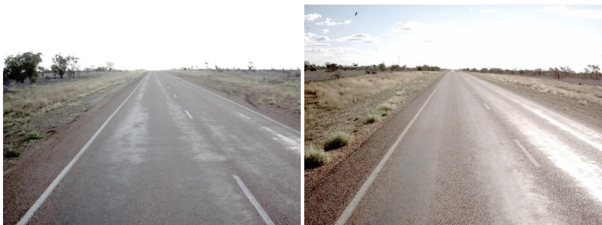
Figure 5.4: Road Section 13E – chainage 26.7 km to chainage 27.6 km
