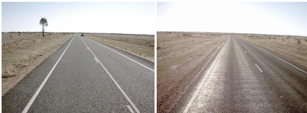
Figure 5.1: Road Section 13B – chainage 100.3 km to chainage 108.0 km (good vs poorer sections)
