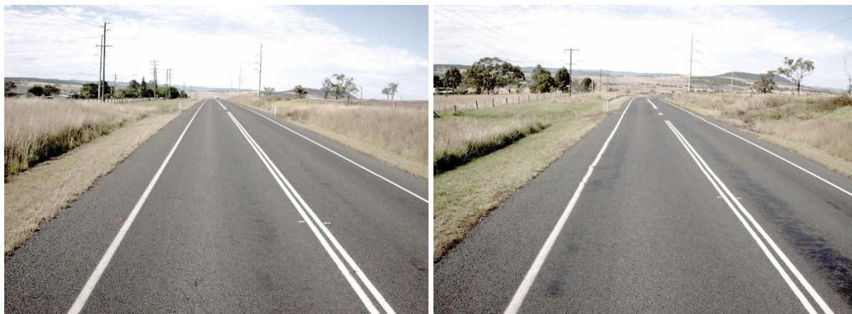
Figure 5.17: Road Section 22B – chainage 22.2 km to chainage 22.9 km
