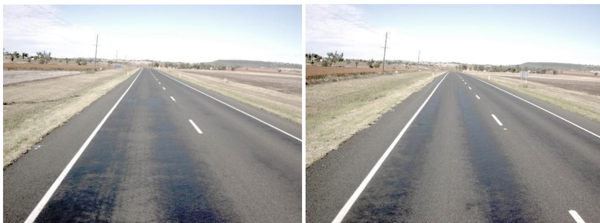
Figure 5.14: Road Section 22B – chainage 15.3 km to chainage 16.0 km
