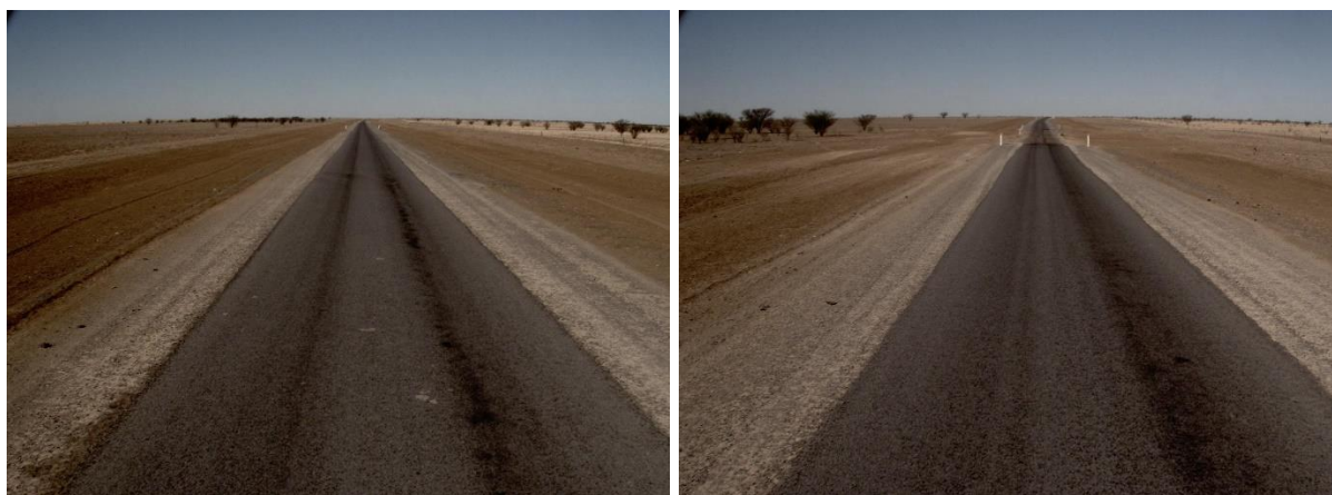
Figure 5.28: Road Section 5803 – chainage 18.7 km to chainage 20.1 km
