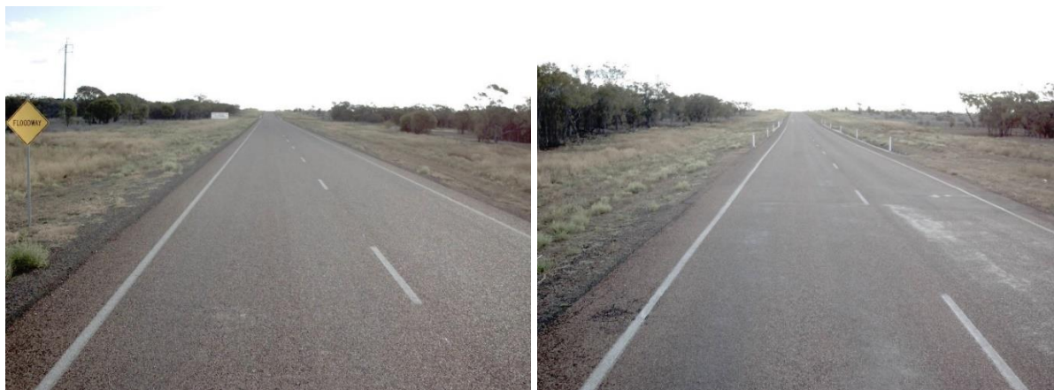
Figure 5.3: Road Section 13E – chainage 24.2 km to chainage 26.6 km
