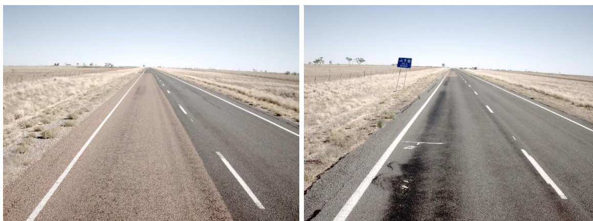
Figure 5.6: Road Section 13G – chainage 92.3 km to chainage 97.8 km
