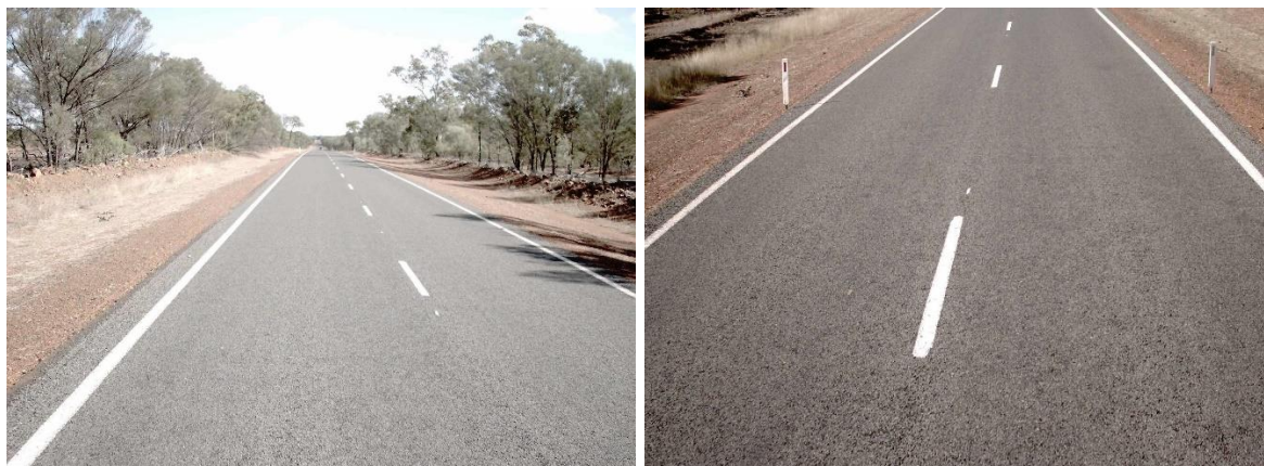
Figure 5.37: Road Section 18G – chainage 35.1 km to chainage 37.2 km
