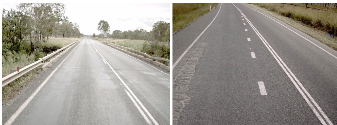
Figure 5.26: Road Section 10E – chainage 98.6 km to chainage 99.7 km
