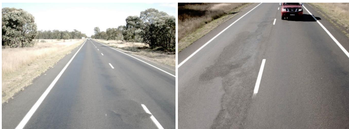
Figure 5.18: Road Section 28B – chainage 70.8 km to chainage 73.1 km
