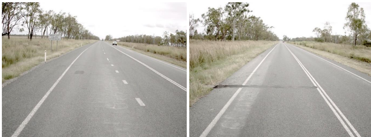
Figure 5.25: Road Section 10E – chainage 97.7 km to chainage 98.6 km
