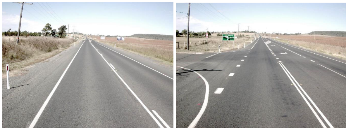
Figure 5.16: Road Section 22B – chainage 17.8 km to chainage 18.3 km
