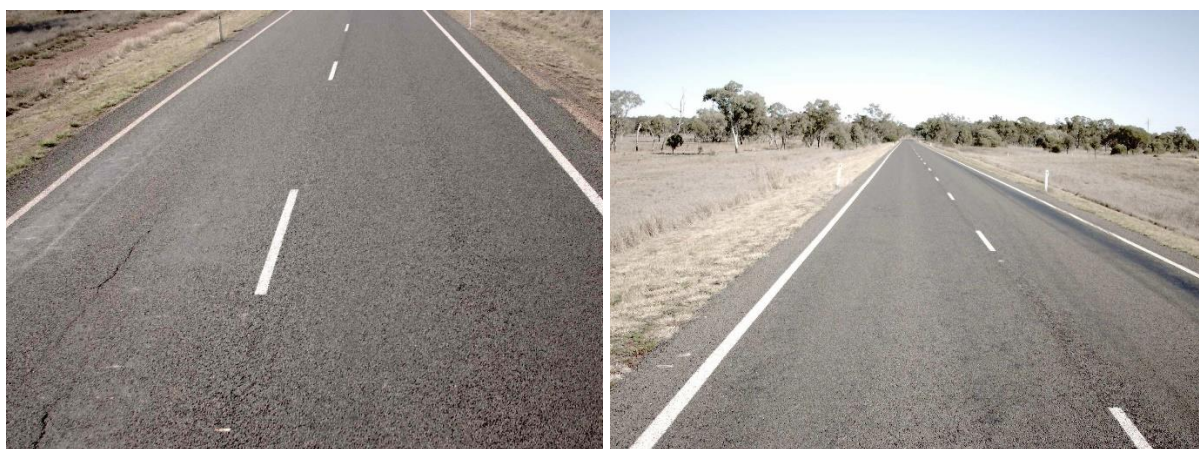
Figure 5.34: Road Section 18F – chainage 47.8 km to chainage 49.9 km
