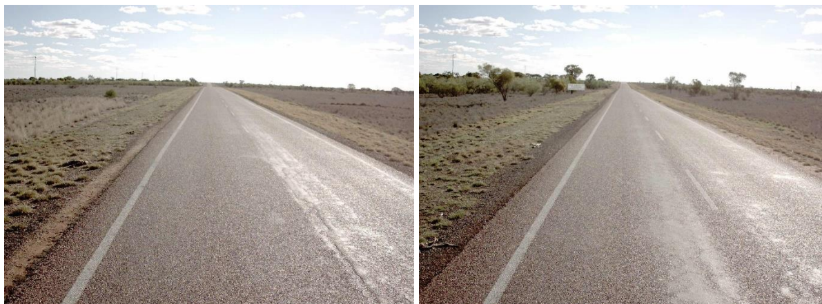
Figure 5.5: Road Section 13E – chainage 32.4 km to chainage 33.9 km
