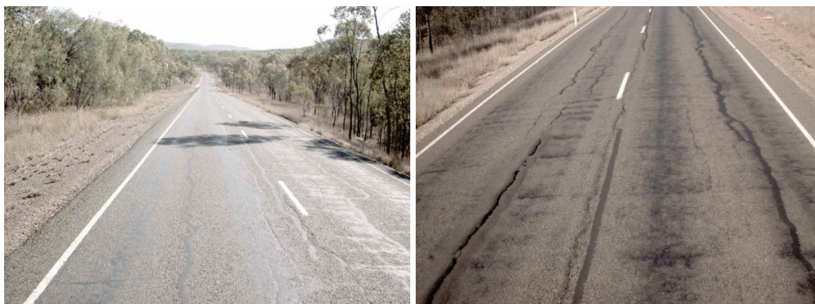
Figure 5.38: Road Section 24E – chainage 51.7 km to chainage 52.9 km
