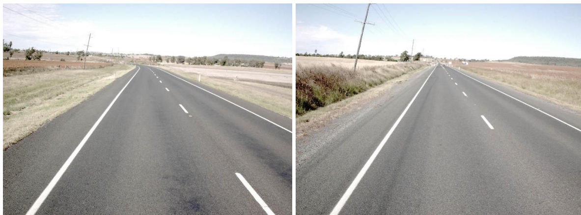
Figure 5.15: Road Section 22B – chainage 16.0 km to chainage 17.8 km
