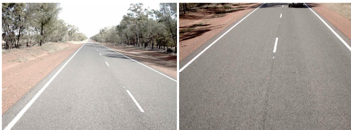
Figure 5.36: Road Section 18G – chainage 11.1 km to chainage 14.3 km
