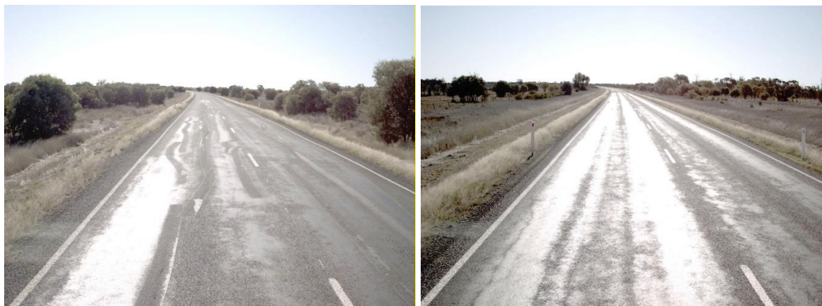
Figure 5.13: Road Section 13B – chainage 45.9 km to chainage 53.3 km
