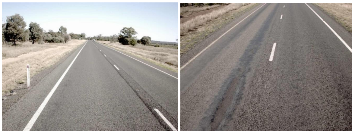
Figure 5.33: Road Section 18F – chainage 42.0 km to chainage 43.2 km
