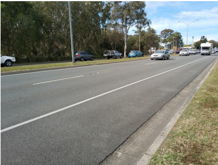
Figure 2.3: Photograph showing the condition of the pavement before installation of ground sensors
