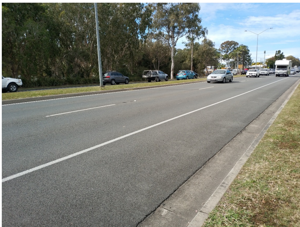
Figure 4.3 Photograph showing the condition of the pavement prior to installation of ground sensors
