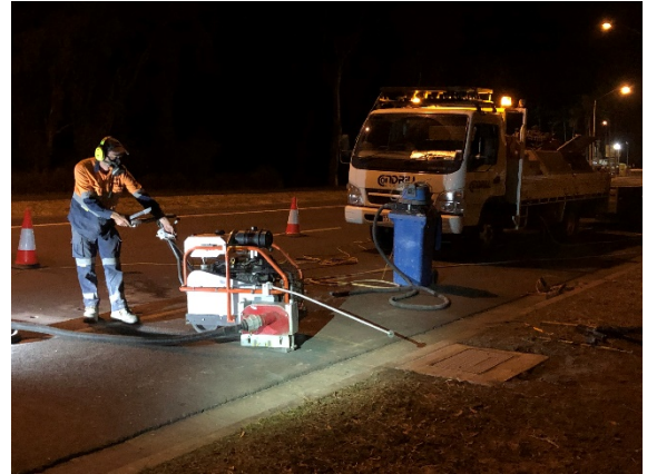
Saw cut for wire to run from sensor to cable pit
