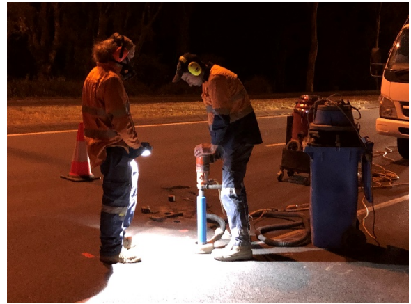
Coring on the pavement surface prior to sensor installation
