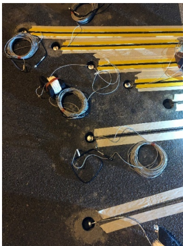
Sensors installed in core holes
