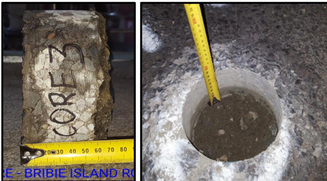
Figure 3.3 Asphalt core sample photos of Site 4 – Bribie Island Road 1
