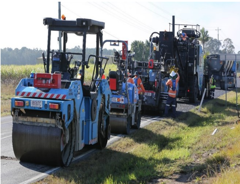
Figure 4.6: Conventional construction equipment
