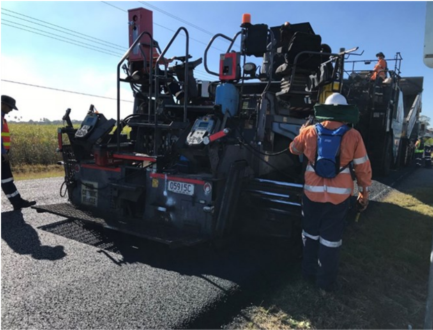
Figure 4.10: Emissions monitoring – note blue backpack on construction worker
