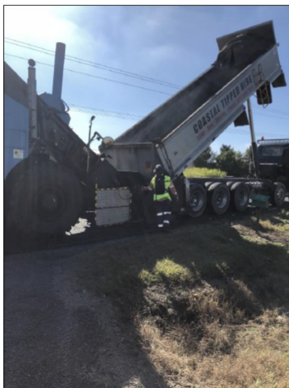
Figure 2: Truck spotting
