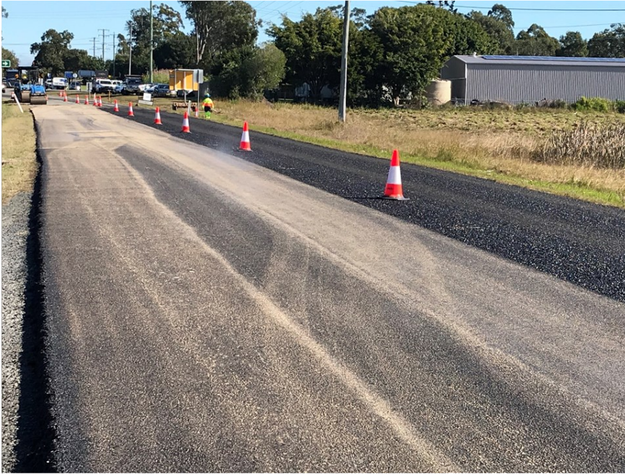
Figure 4.7: Sand grit applied to the surface to improve early-life skid resistance
