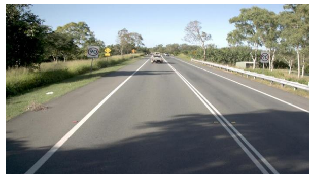
Speed sign 90 and Metal barrier at RHS
