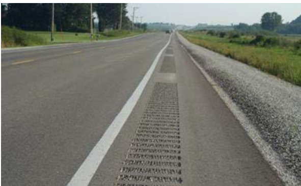
Figure 2.4: Shoulder rumble strips
