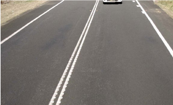
Figure 2.3: Centreline rumble strips
