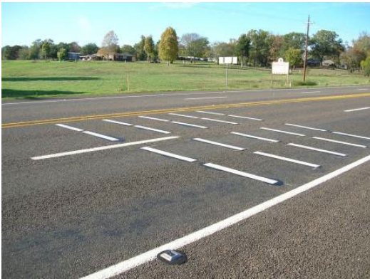
Figure 2.6: Transverse rumble strips
