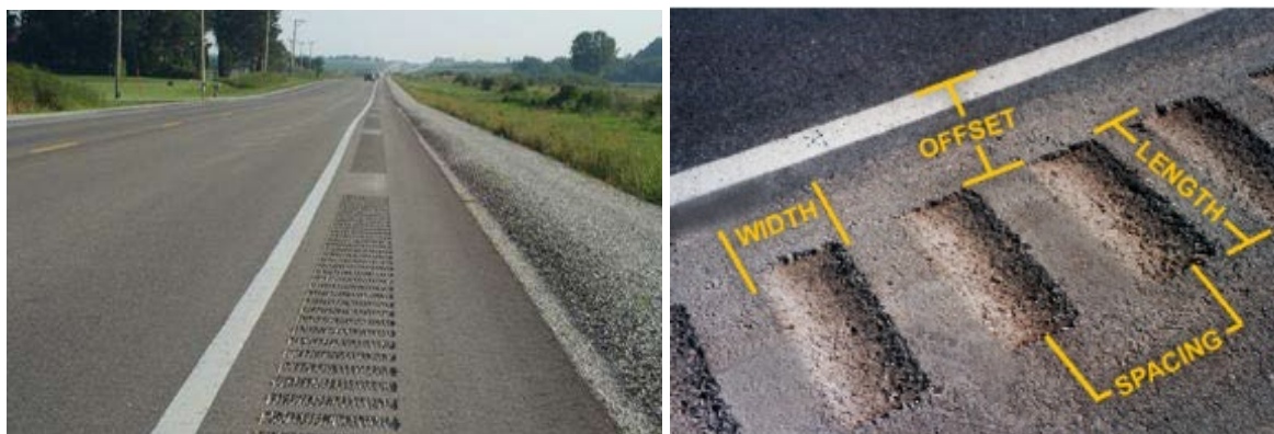
Figure 2.1: Milled rumble strips
