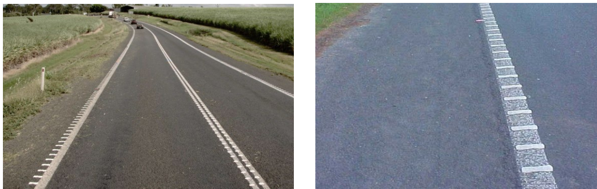
Figure 2.2: Raised rumble strips
