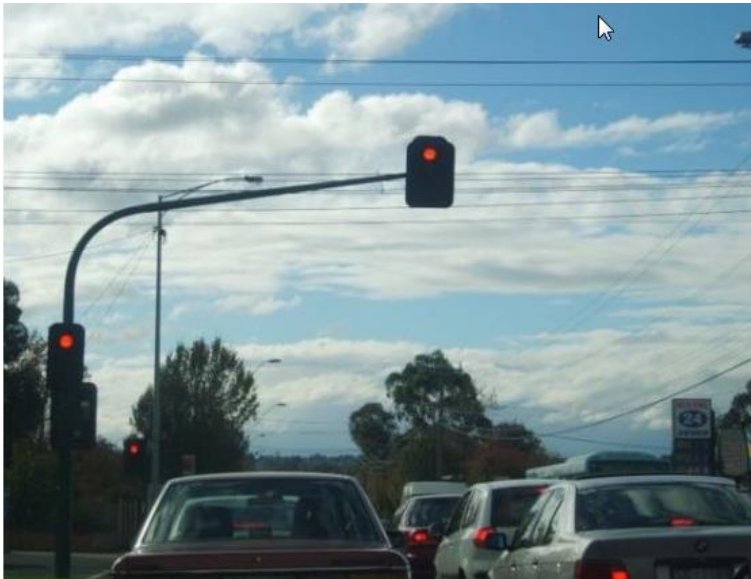
Figure 6.10: Traffic signal displays mounted on a mast arm
