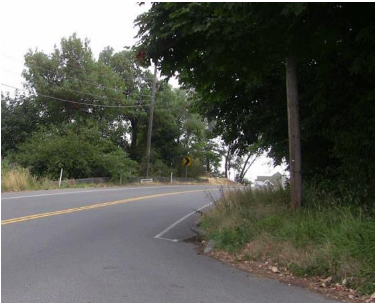
Figure 6.9: Sight distance limited due to intersection being on the inside of a curve and by vegetation
