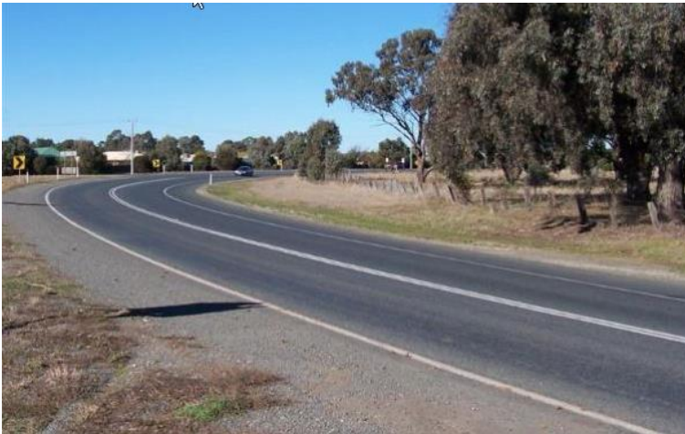
Figure 6.3: Curve widening on shoulders
