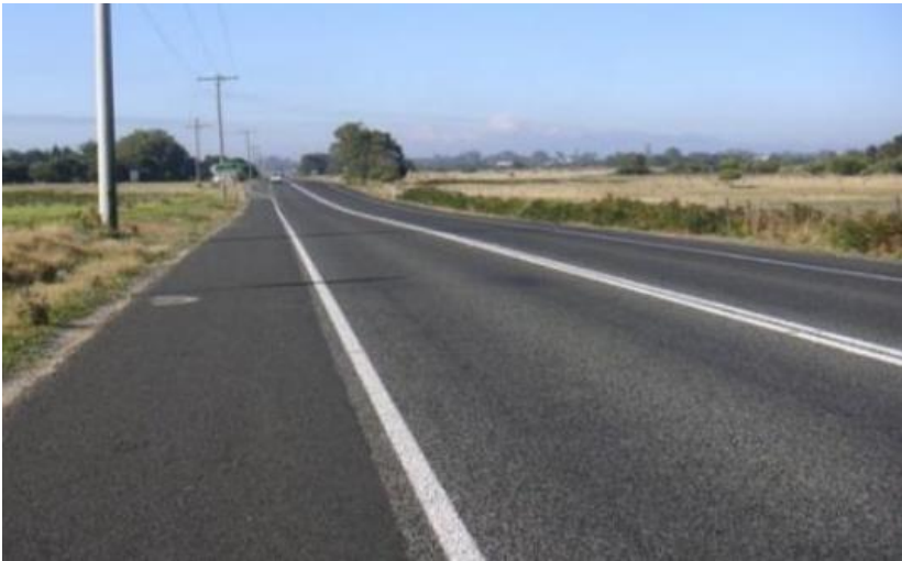
Figure 6.4: Recently sealed shoulder on two-lane road
