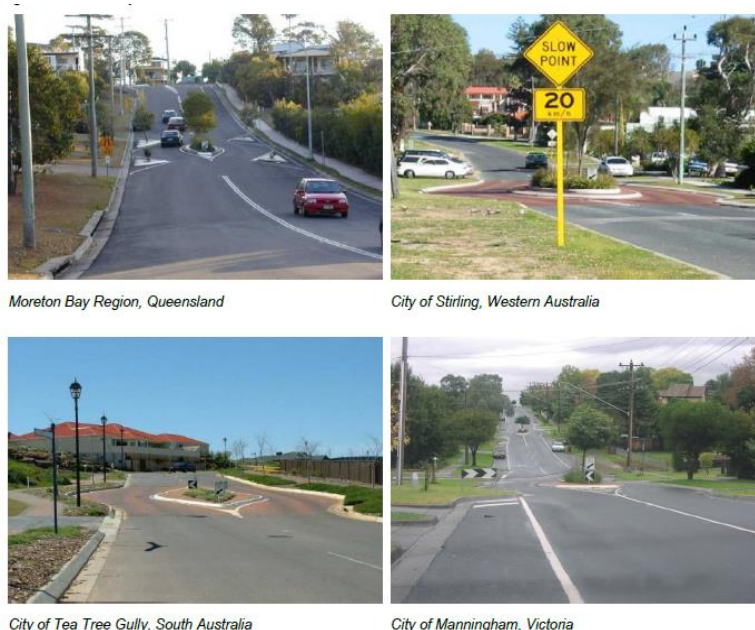
Figure 2.6: Examples of centre blister treatments
