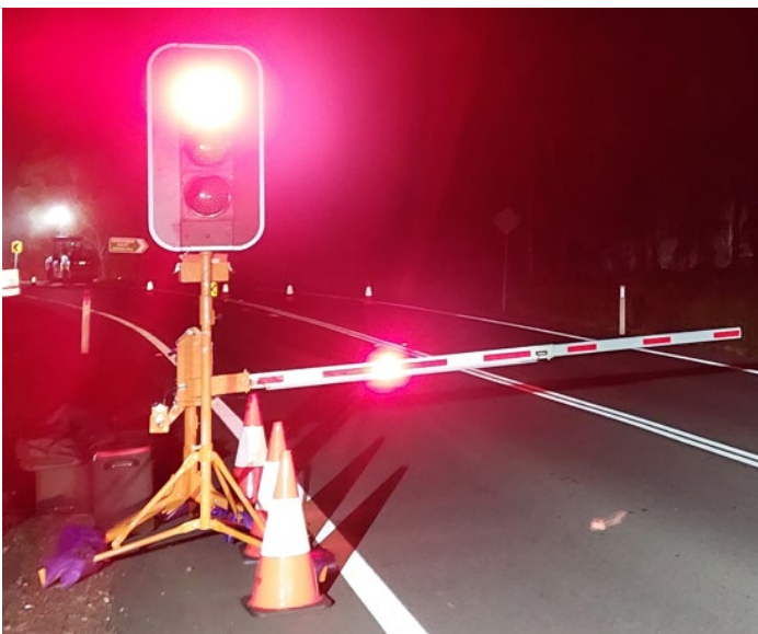
Figure 4.3: Combined portable traffic signal and PTBB (photo taken at the project site)
