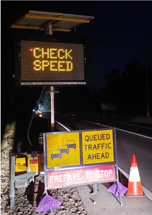
Figure 4.2: VMS (photo taken at the project site)
