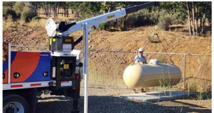
Finishing touches. Work finalized the newly constructed Karuk Judicial Building, Yreka CA.
