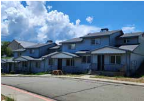
Yreka Completed Siding
