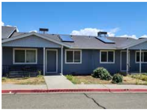
Yreka Completed Siding
