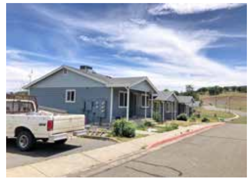
Yreka Completed Siding
