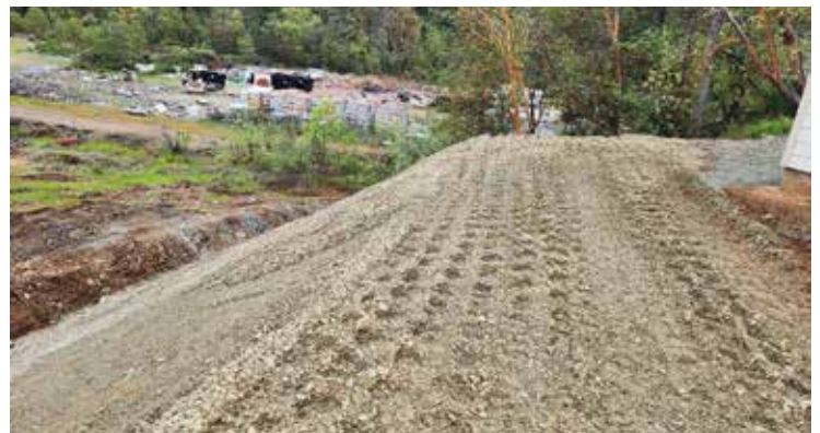
Retaining wall created to stabilize construction of new Medical & Dental clinics in Happy Camp, CA
