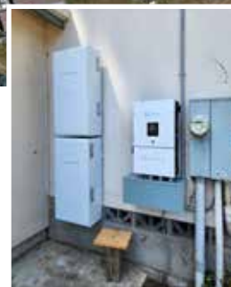
Above: Orleans Elder Units Right: Typical Battery Installation
