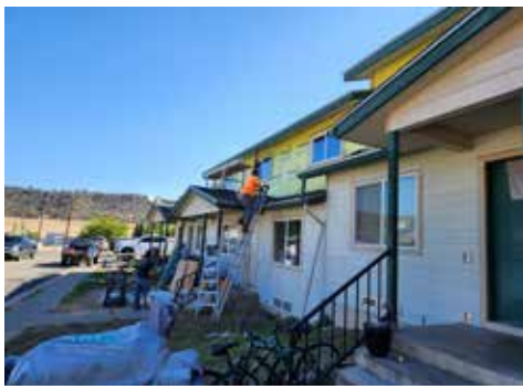
Yreka Work in Progress
