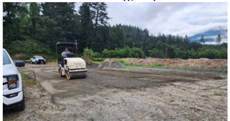
Ground work for building pad to support refrigeration Conex at the Tishaniik Farm, Orleans CA.
