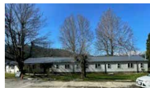
New roof on Karuk Tribe's Klamath River Resort Inn
