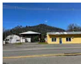
Site of new Mechanics, Maintenance and Laundromat in Happy Camp
