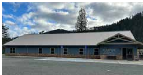
Dental Facility part of Medical Complex in Happy Camp is now open
