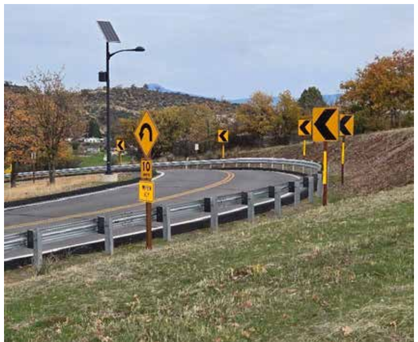
New guardrail & curve warning signs
