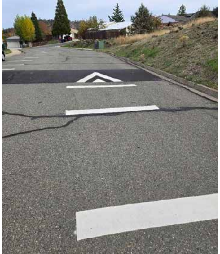
New speed hump and striping
