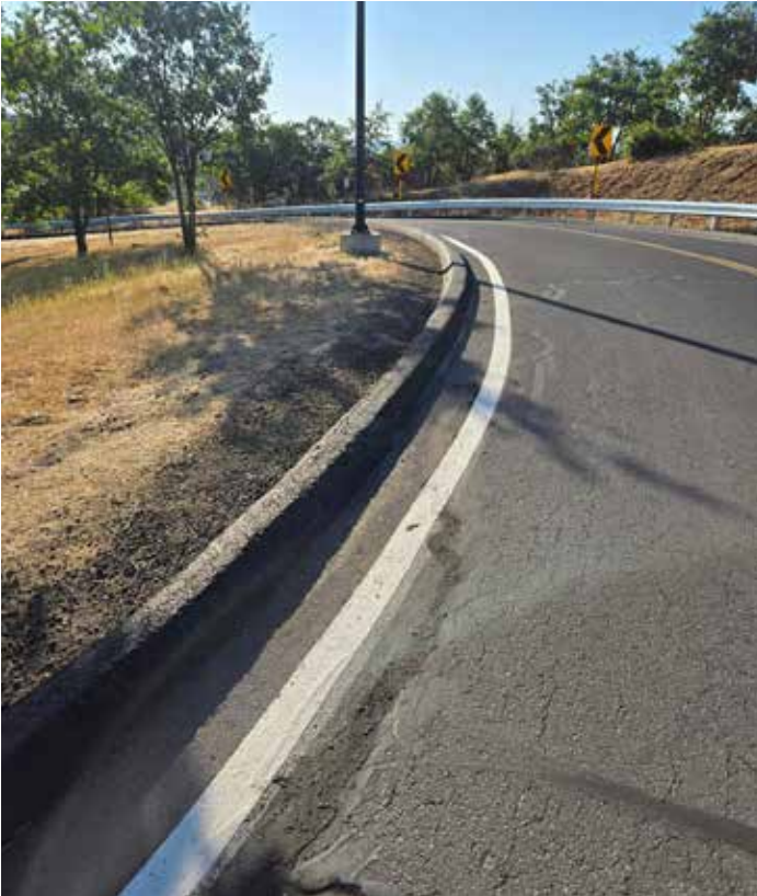
New curb, guardrail, signs & striping
