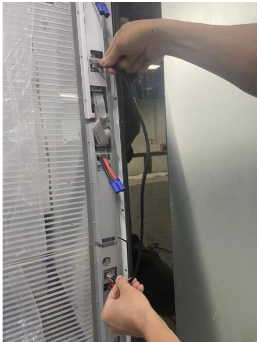
6.3 LED film signal cables connection, signal input from top.
