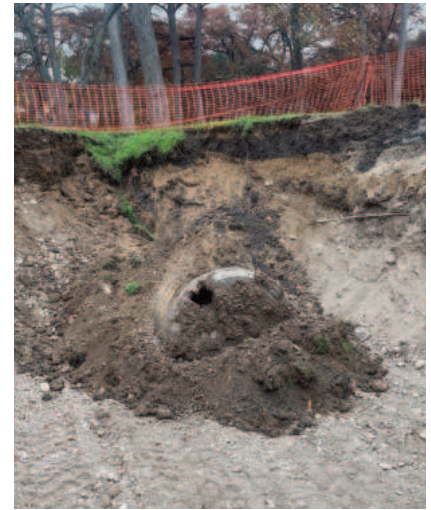
Figure 8. Installation was generally smooth except for sticky clays
