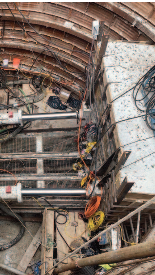
Figure 5. RCP hydraulic joint configuration
