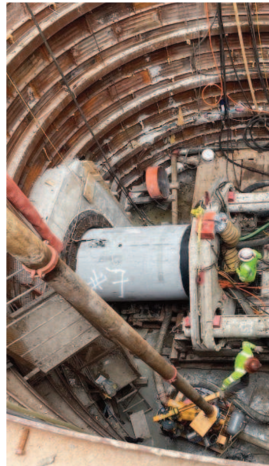
Figure 6. Jacking frame and casing pipe within installation shaft
