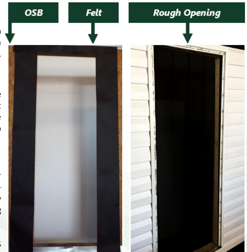
Figure 1: OSB & Felt. Black felt is overlapping the edges of the rough opening. Figure 2: Rough opening.
