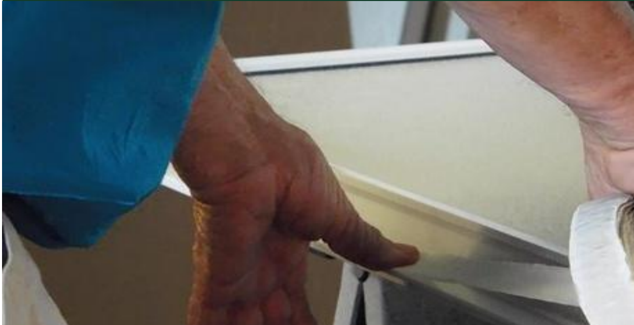
Figure 3: Sealing tape being applied.
