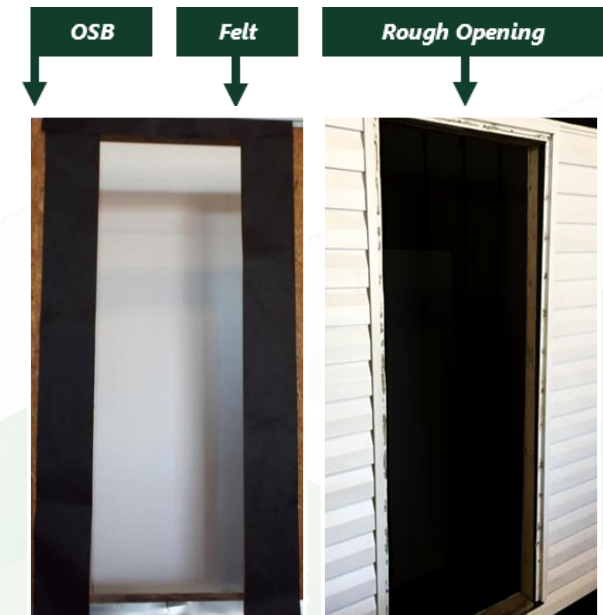
Figure 5: OSB & Felt. Black felt is overlapping the edges of the rough opening.
