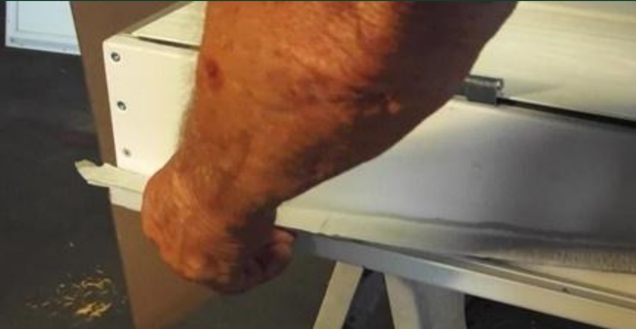
Figure 8: Sealing tape being applied.
