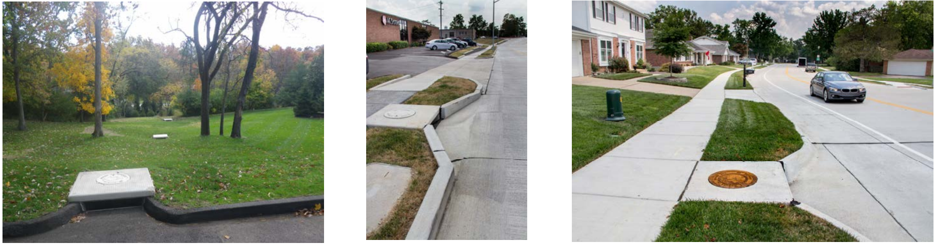
Single curb inlet with asphalt curbs Single curb inlet with concrete vertical curbs Single curb inlet with concrete mountable curbs
