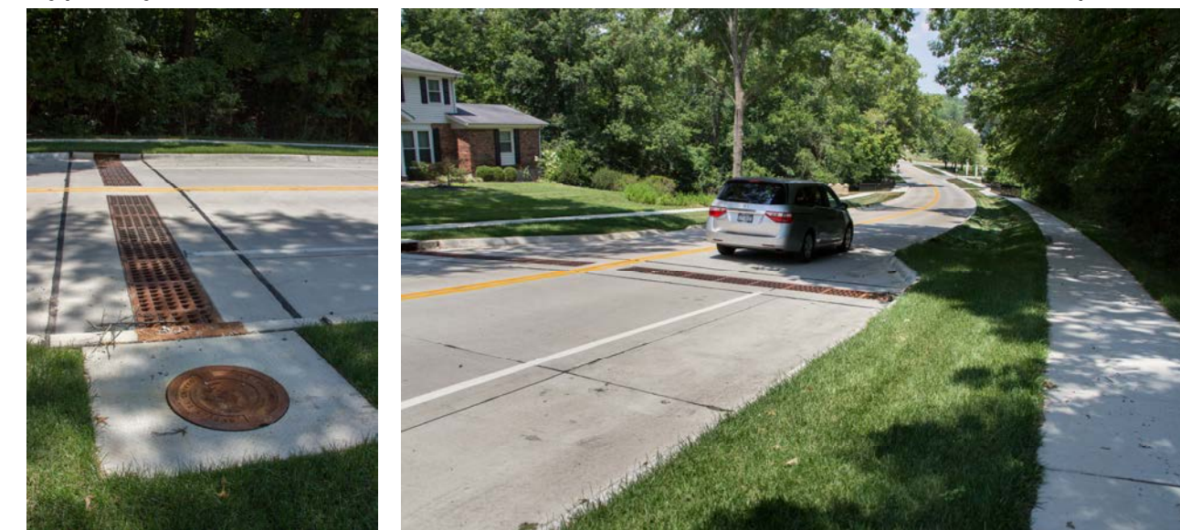
Typically one end of a trench drain has a manhole, as seen in the left picture
