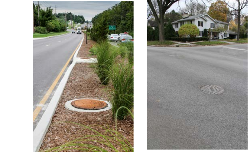
Manhole (in foreground) Manhole in street
