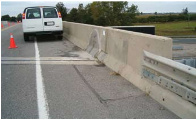
Fig. 1: Cores were taken from the barrier wall of the Chatham Bridge in Chatham, ON, Canada
