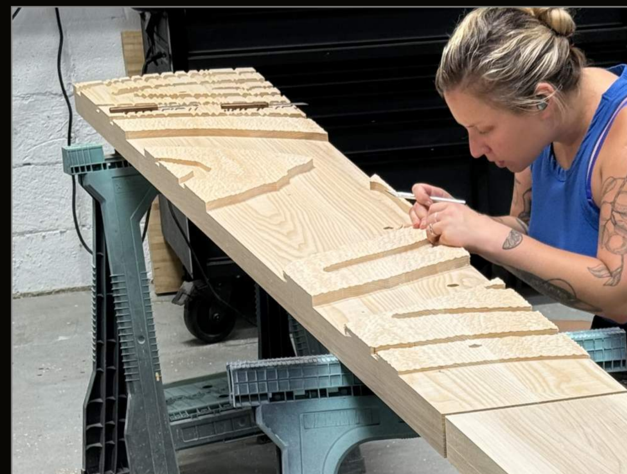
Center The full-scale visual mock-up panel receive patterning before raised wood elements are placed by hand into the recessed grooves shown here.
