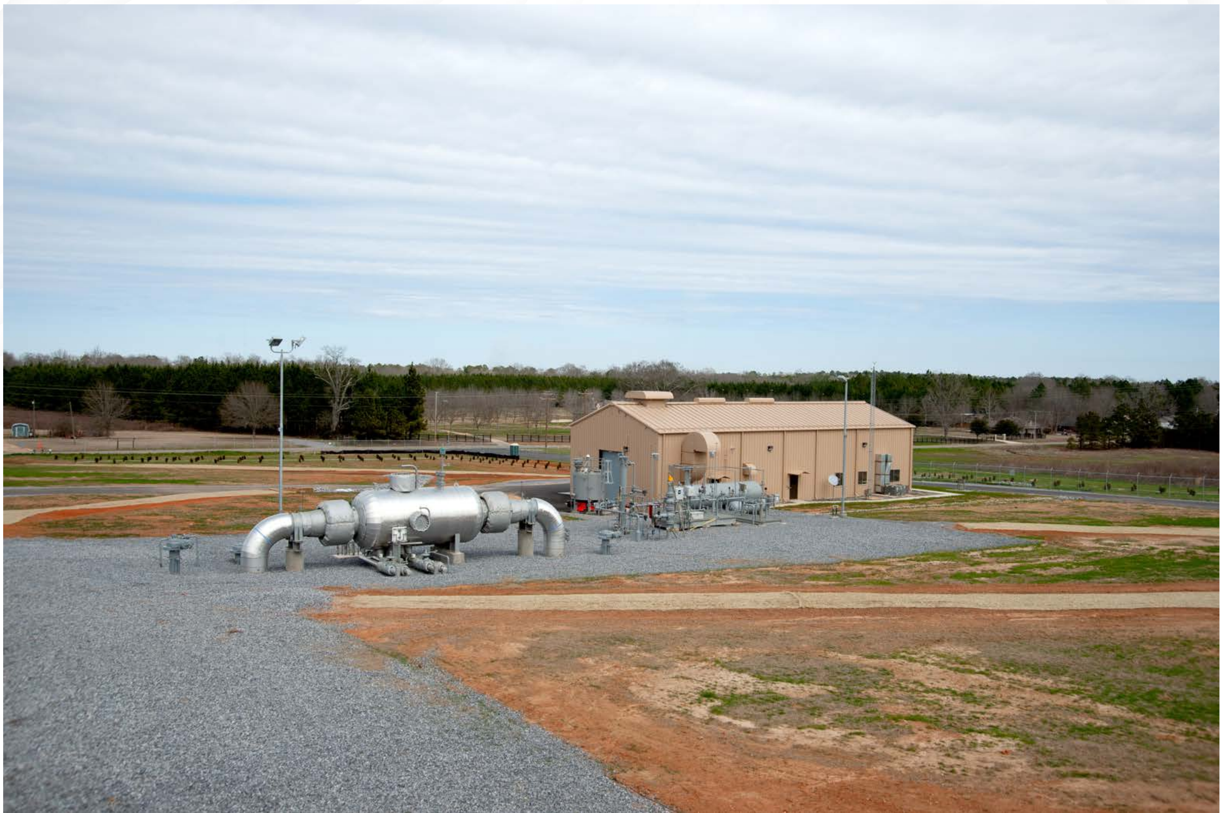
Forrest Compressor Station
