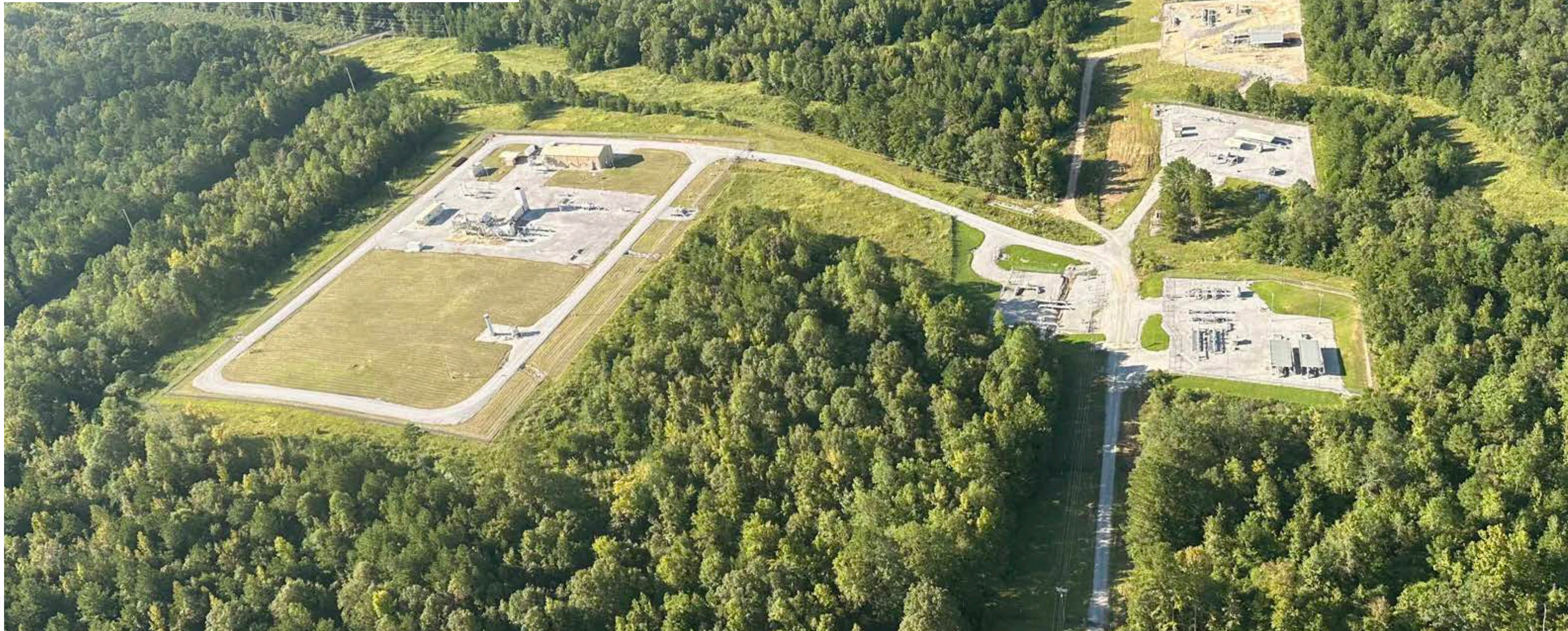
Jasper Compressor Station
