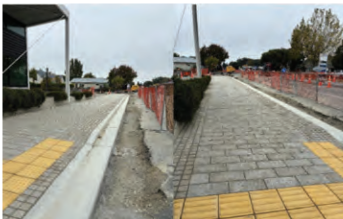
New pavers on Gerald Street
