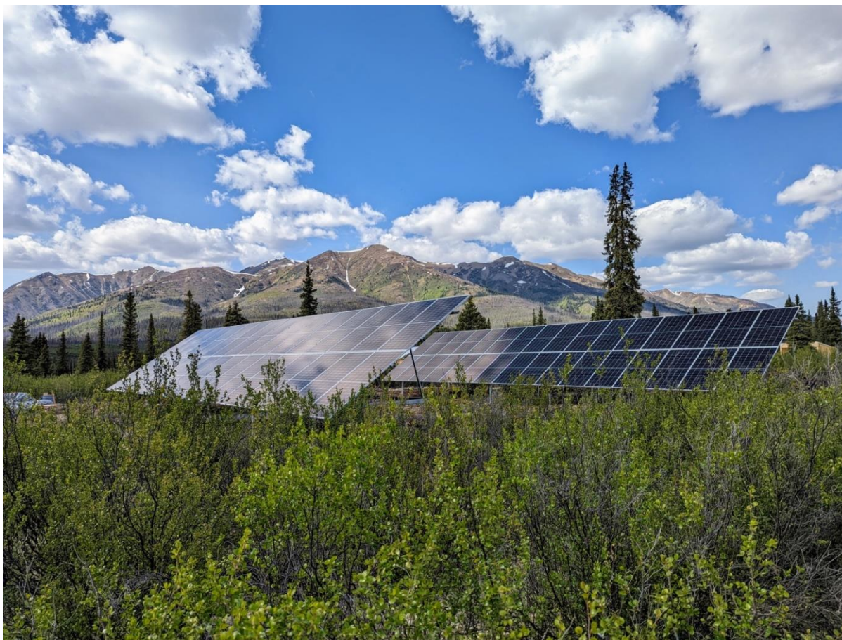
Solar panels in position at Snowline's newly built Forks Camp. Designed by Solvest Inc. the 27-kW hybrid-solar generator system is among the first of its kind to be used to power a remote exploration camp in Canada.
