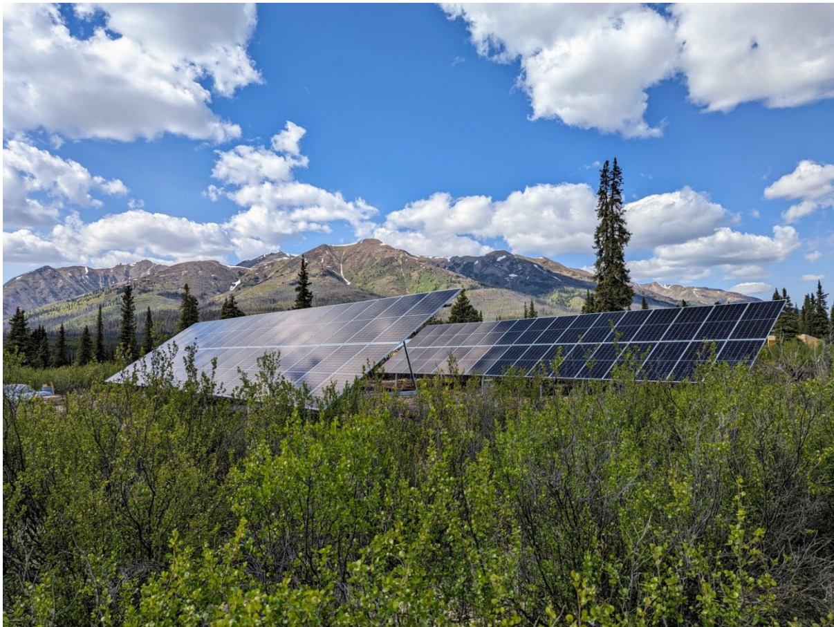
Solar panels in position at Snowline's newly built Forks Camp. Designed by Solvest Inc. the 27-kW hybrid-solar generator system is among the first of its kind to be used to power a remote exploration camp in Canada.
