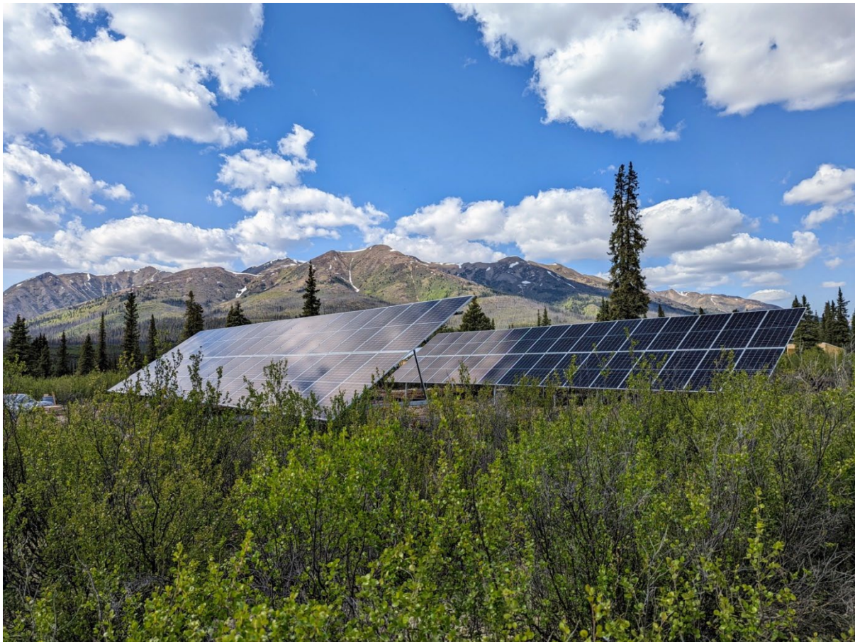
Solar panels in position at Snowline's Forks Camp. Designed by Solvest Inc. the 27-kW hybrid-solar generator system is among the first of its kind to be used to power a remote exploration camp in Canada.
