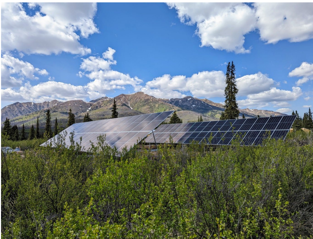
Solar panels in position at Snowline's Forks Camp. Designed by Solvest Inc. the 27-kW hybrid-solar generator system is among the first of its kind to be used to power a remote exploration camp in Canada.
