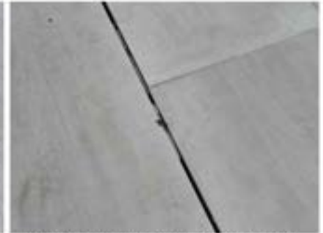
Tile Separation - Grout Deterioration
