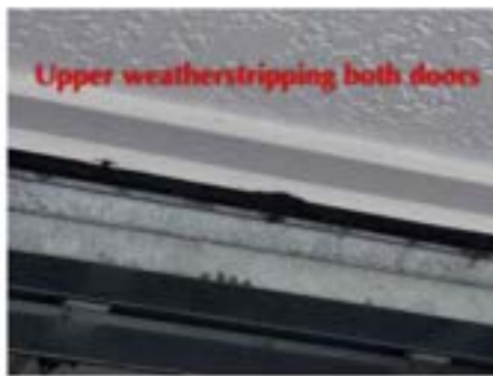
Damage to garage door weatherstripping
