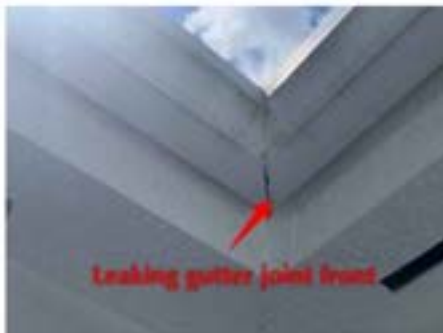
Leaking joint
