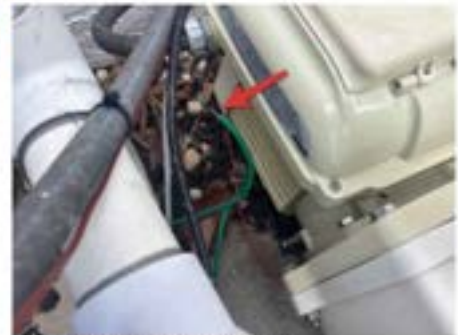
Disconnected Bond Wire
