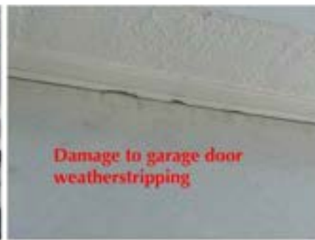
Upper weatherstripping both doors
