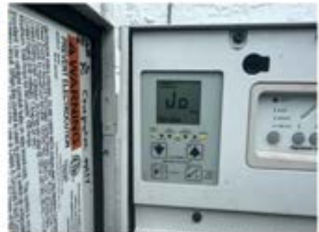
Service Indicator for Salt Chlorinator
