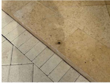
Remnants of rusty screen enclosure mounting bolts
