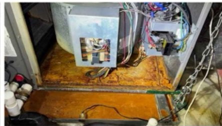
Rust & Deterioration
