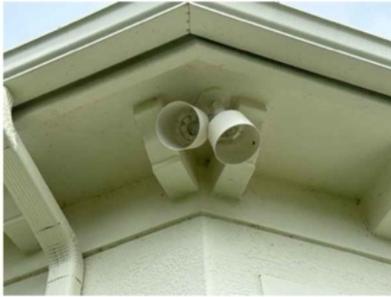
Left Rear Corner
