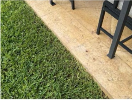
Remnants of rusty screen enclosure mounting bolts
