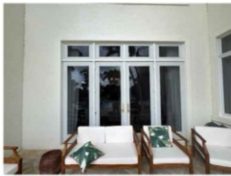
Rear Picture Windows
