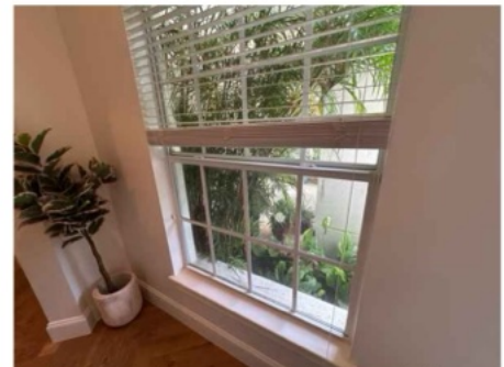
Left side hallway, single hung window
