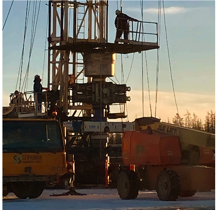
Shown Right: K-BOS added to the stack as an additional barrier where stack height is not a limiting factor.
