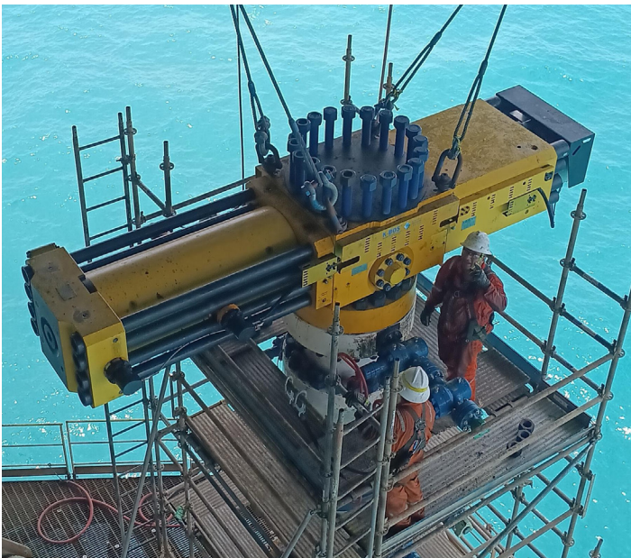
Shown Left: K-BOS added to a BOP stack as a replacement for the drilling cross flow spool.
